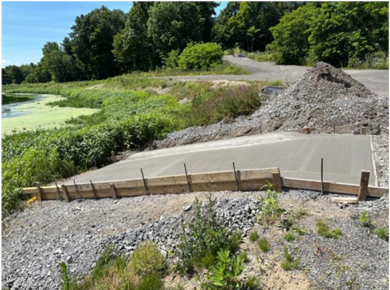
Figure 2: Lagoon Cell 1 Ramp
